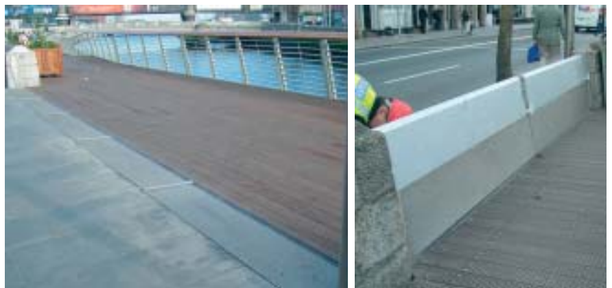
The Dutchdam-Duplo 80 as applied in 8 places in the city centre in Dublin, Ireland, in lengths of 5, 8 and 12 metres.
